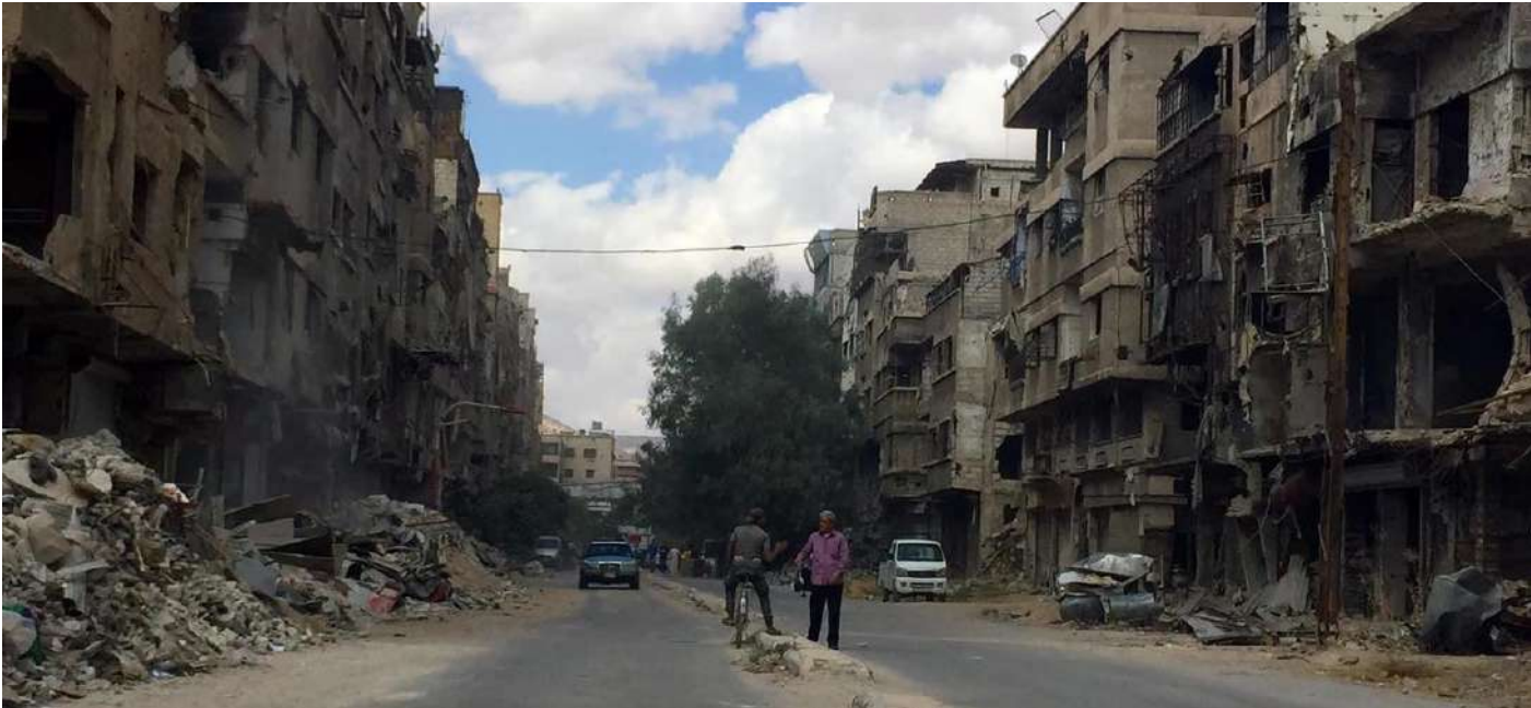
A street in Yarmouk camp after its destruction
